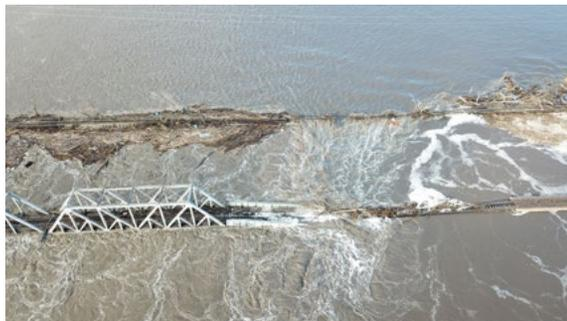
The Platte River caused widespread flooding, including this track washout south of Bellevue, Nebraska.
